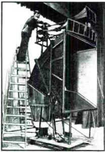
(I'hoto-W. E. Shrage) e speaker for Berlin theatre capable of 1,000 watts is largest hi-fi unit in world. hs a ton and reproduces faithfully from 10,000 down to 40 cycles. Movable handling weighs
